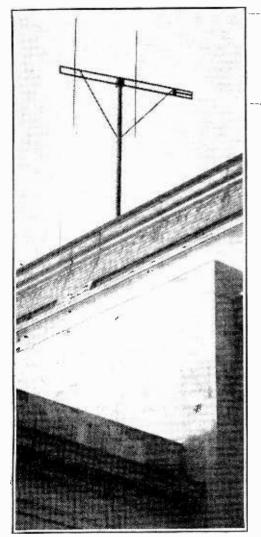
EARLY all the special aerials now in use for television reception are what are known as dipoles, or some variation of this arrangement, the total length of the aerial being approximately half the length of the wave used for transmission.
