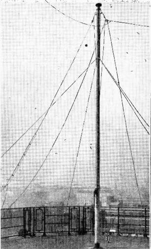
The television aerial with matching section for a low-impedance feeder can be seen to the left of other aerial systems erected on the roof of *The Wireless World* laboratory.
