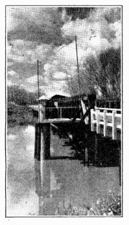
RADIO FLOOD GAUGE. As a precaution against avoidable repetition of recent dis-asters due to floods, the authorities in California have installed automatic wireless transmitters, actuated directly by water gauges which measure river levels, at certain of the more remote danger points. Dry batteries are used for both HT and LT, while the receivers are put into operation at pre-determined hours by time-switches.
