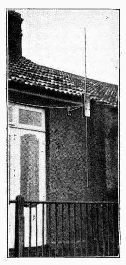
TELEVISION AERIAL. A practical interpretation of a di-pole television aerial with centre-connected feeder as shown in Fig. I(a) on page 506 of this issue.
